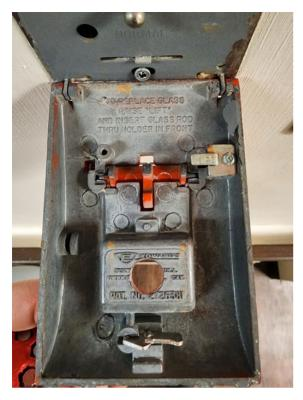
Raise the "lift" tab, insert the glass rod thru the holder in the front cover on the other side.
