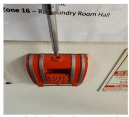
Insert Flat head Screwdriver in top and turn clockwise
