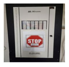
A.C ON" should be the only thing always lit up \*To RESET after a Fire Drill-Press "SYSTEM RESET" button
